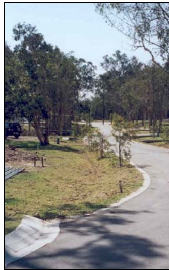
Figure 10. Example of flush kerbing and grass swales, Brisbane, Qld. (Photograph: Department of Environment 2002.)
