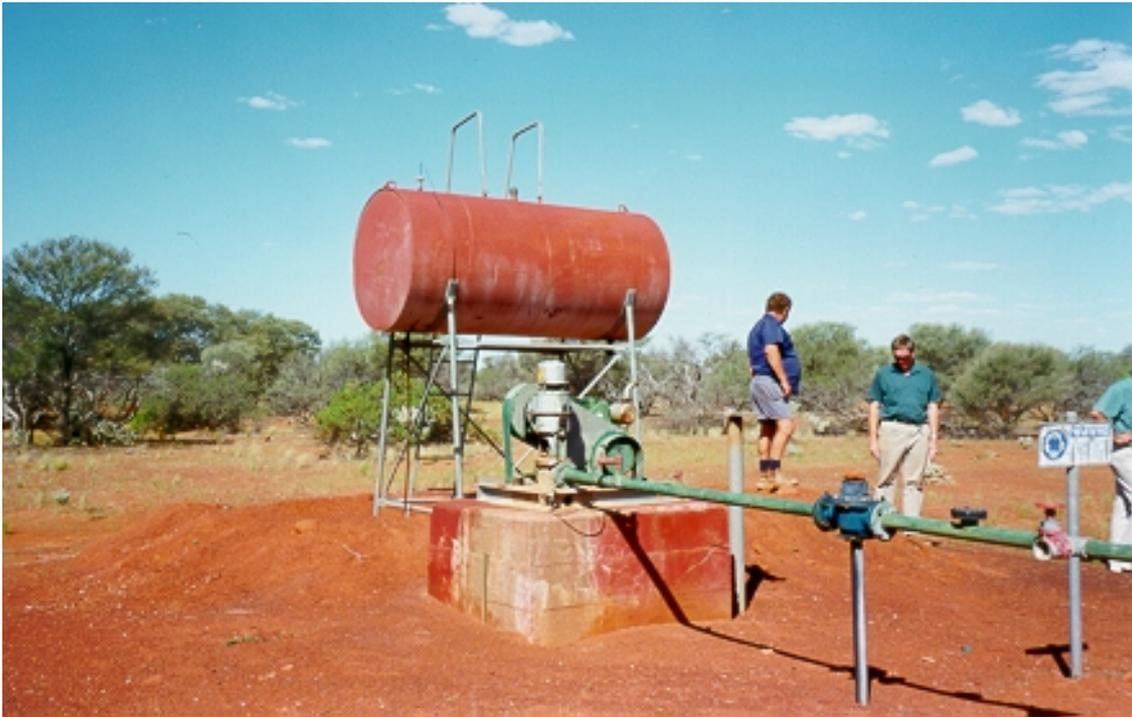
**Plate 2. Production bore 5/85 and elevated fuel storage tank. Similar to production bore 12/85.**
