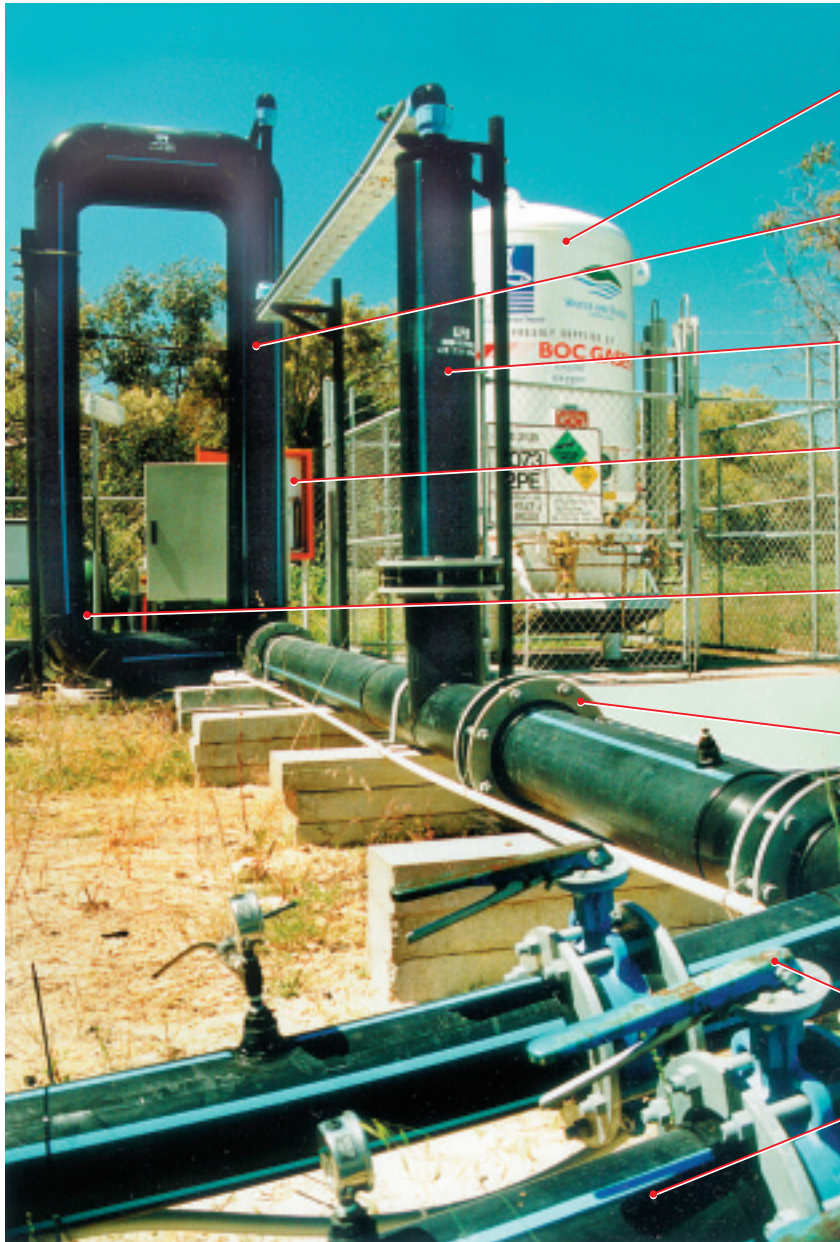
Figure 3: The oxygenation plant used in the 1998/99 trials
