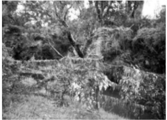
Figure 1: Debris caught on a conventional star picket fence during the Moore River floods 1999. K. Griffin
