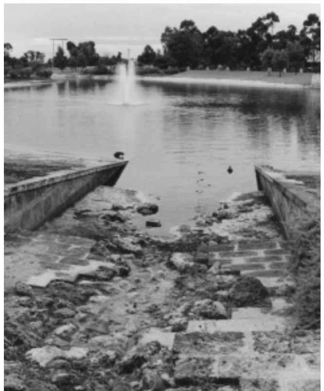
A stormwater drain enters a significantly modified wetland in an urban environment. Stormwater drains are a common sight in many urban wetlands.
