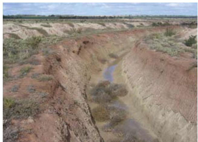
The silty soils of the Pithara upstream drain have low permeability and erode quite easily. The channel is only 2 years old.
