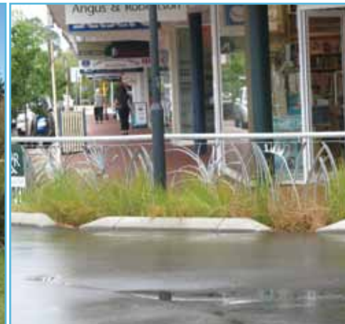
Roadside biofilter retrofit, Busselton CBD
