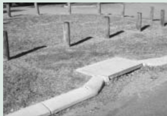
Figure 4. Remove grass cuttings from roads and paths to ensure they do not enter the stormwater system. (Photograph: South East Regional Centre for Urban Landcare.)
