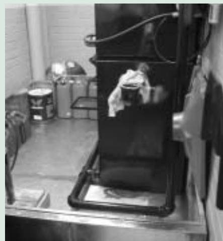
Figure 1. Green Stamp automotive premises, Balcatta. Correct storage of fuel and other chemicals in a bunded area. (Photograph: Department of Environment.)
