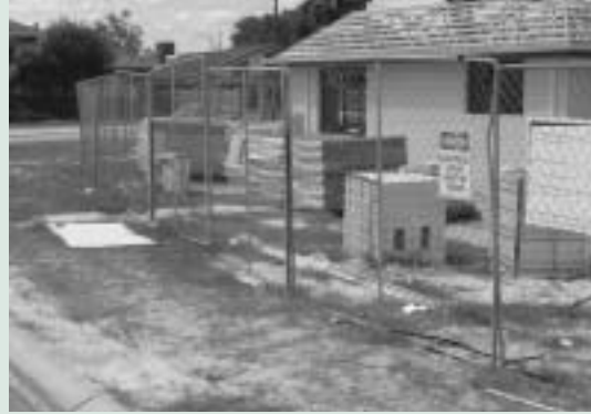
Figure 2. Site fencing for litter containment and security. (Photograph: Clean Site, Keep Australia Beautiful Council WA.)
