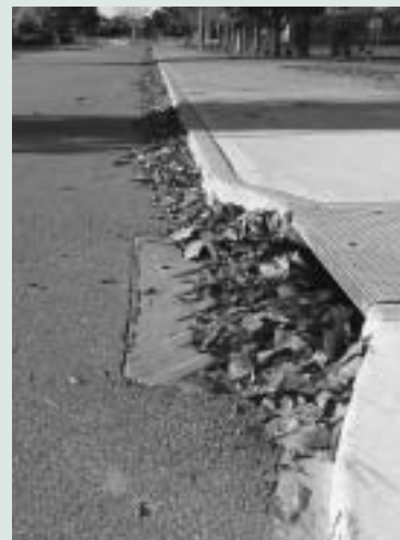
Figure 3. Deciduous leaves can release a large amount of nutrients into receiving water bodies. (Photograph: Eastern Metropolitan Regional Council.)
