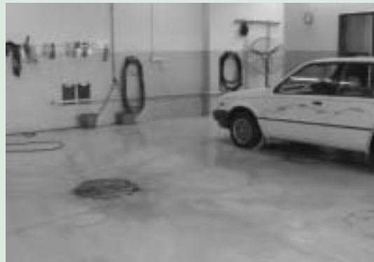
Figure 2. Green Stamp automotive premises, Balcatta. Vehicle wash-down area, with collection drain for wastewater treatment. (Photograph: Department of Environment.)
