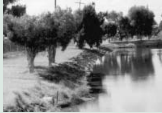
Figure 2. Sediment cleared from a stormwater compensation basin and spread on the banks. Mill Street Compensation Basin, Welshpool. (Photograph: Department of Environment.)
