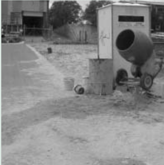
Figure 3. Cement mixer wash-water runoff and sand on the road. (Photograph: Clean Site, Keep Australia Beautiful Council WA.)
