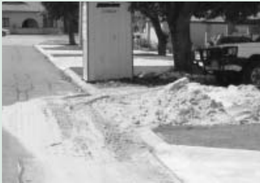
Figure 5. Sand stockpile erosion onto a road. (Photograph: Clean Site, Keep Australia Beautiful Council WA.)
