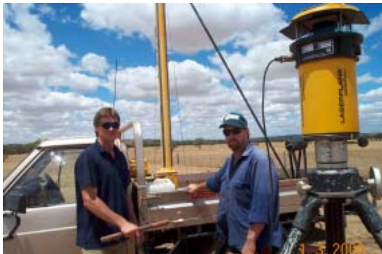
Plate 4 Constructed grade banks being surveyed
