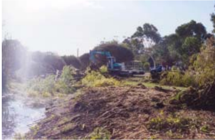
Plate 6 Willow trees being removed prior to revegetation with native plants
