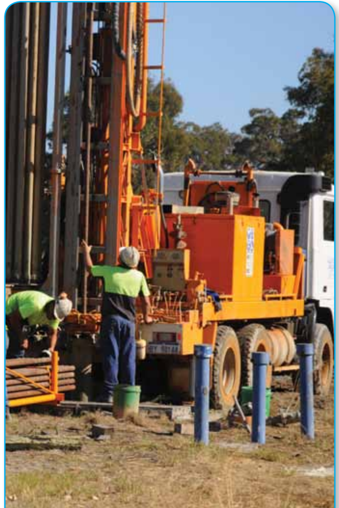
Drilling for groundwater investigation.
