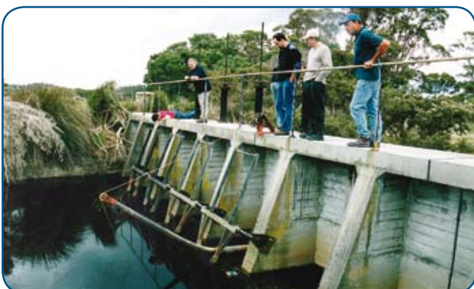
← Review of Lake Manarup penstocks (floodgate) by members of the drainage management committee (Photo: Department of Water)
