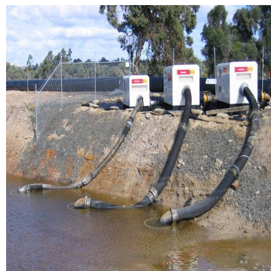
Trial diversion site - Buckingham
