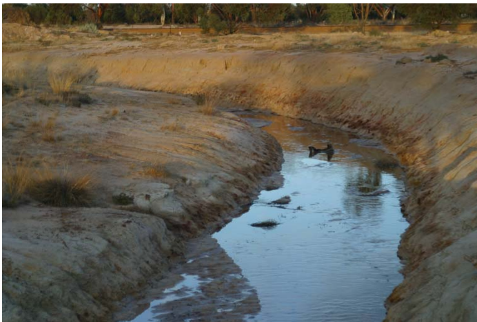
Figure 1.1 Photograph of a drain at Narembeen in the wheatbelt of Western Australia
