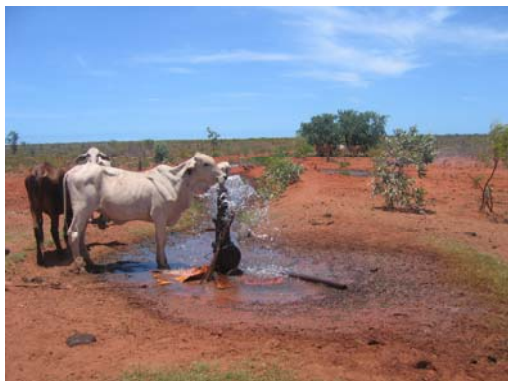
An uncontrolled artesian bore.
